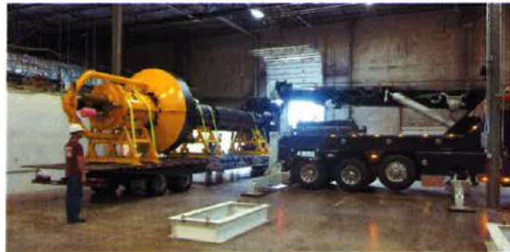
Figure 6 Crane Loading of the Buoy
